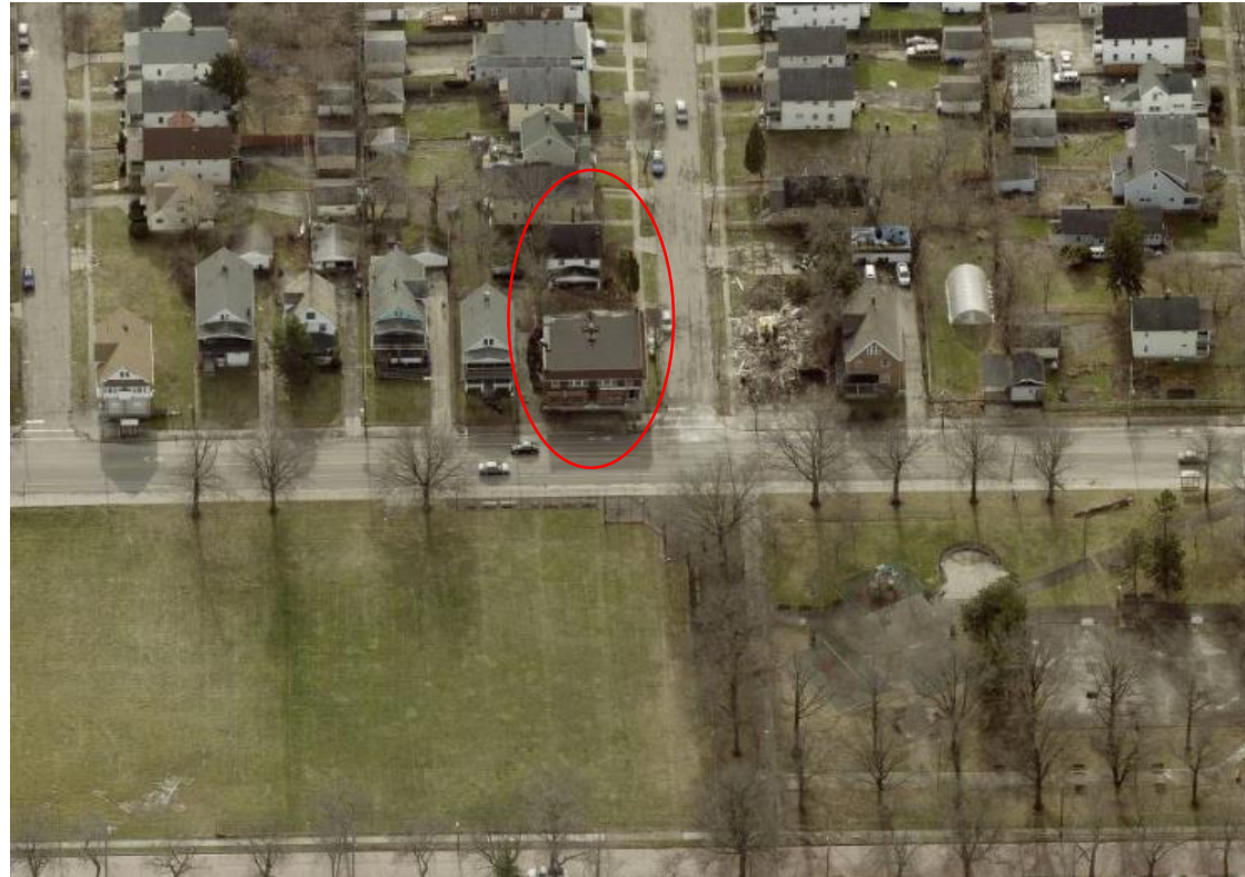
Properties at 13800 Harvard Ave before demolition of the front structure.
